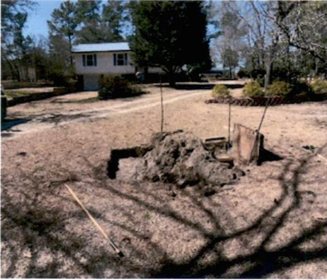
Overall View of Septic Tank
