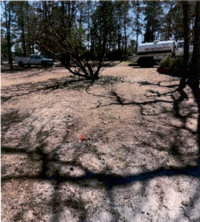
Back Side View of Septic System and Vegetation Over Drain Field.
