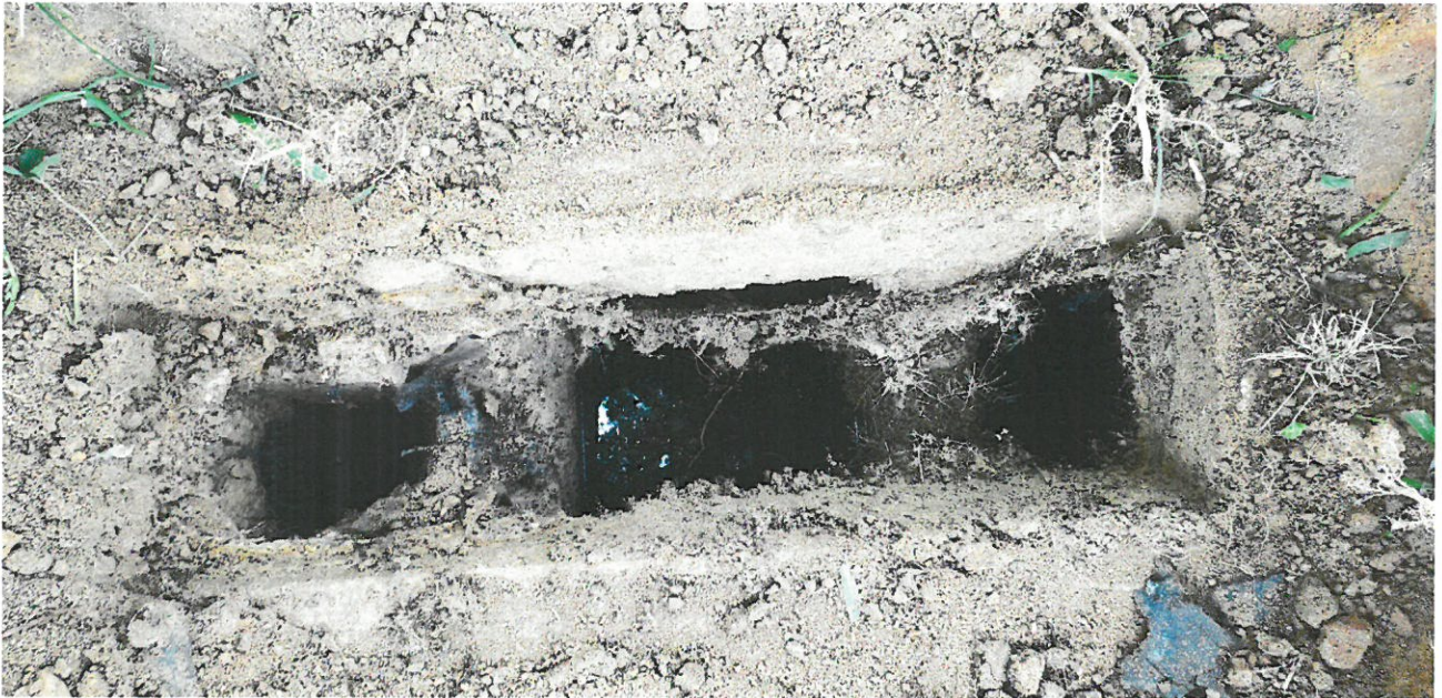
View of Septic Tank Outlet End
