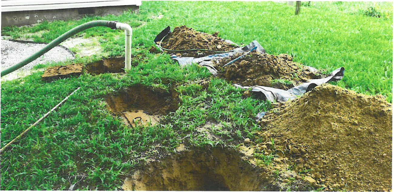
View of Septic Tank Pumping
