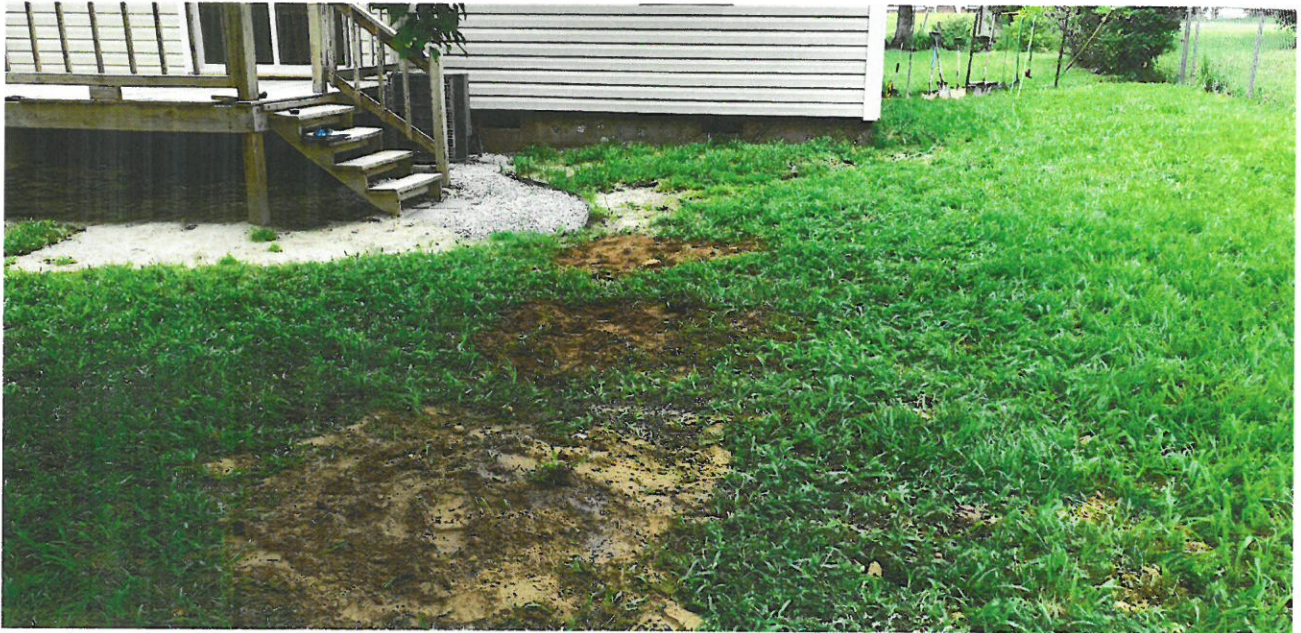
Excavations Filled and Site Cleaned
