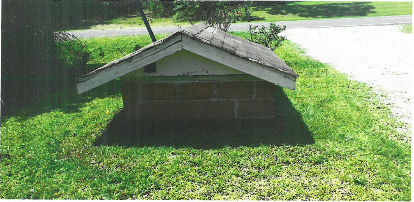
View of Well House Structure Covering Well Head
