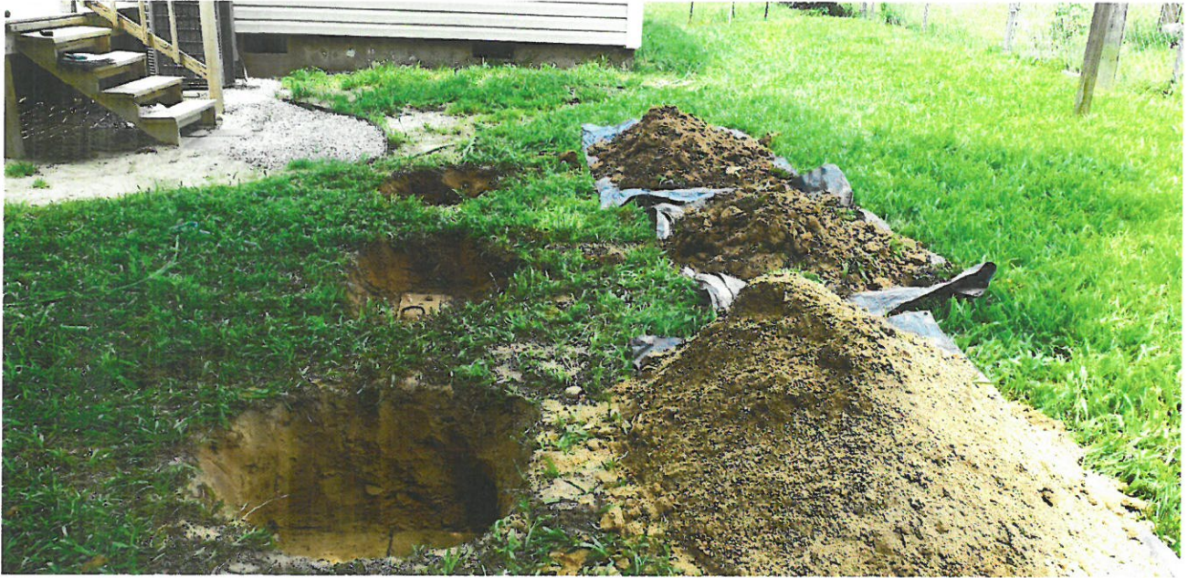
View of Distribution Box Location
