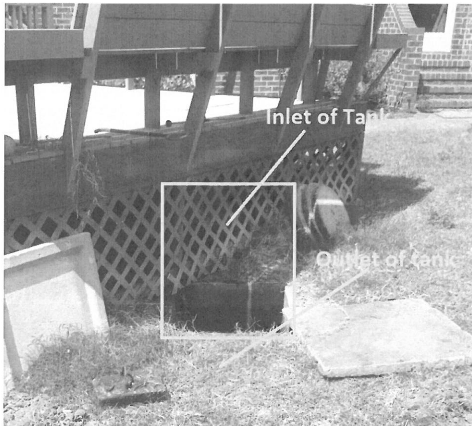
Figure 1. Septic tank (partly beneath deck)
