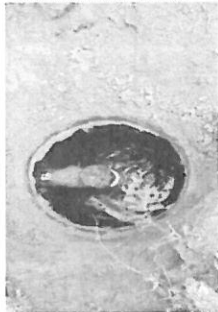
TANK OUTLET & TEE
