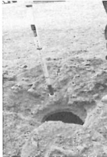
SLUDGE LEVEL INLET
