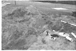
us Repair SR 1271 Shue Rd 6
