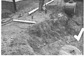
us Repair SR 1271 Shue Rd 6
