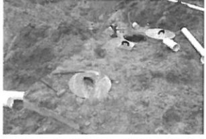
us Repair SR 1271 Shue Rd 6
