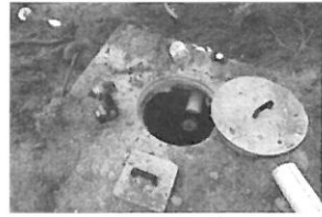
us Repair SR 1271 Shue Rd 6
