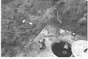
us Repair SR 1271 Shue Rd 6
