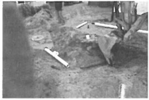
us Repair SR 1271 Shue Rd 6
