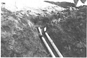
Repair Tank 4-16-19 140 Poi
