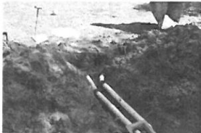
Repair Tank 4-16-19 140 Poi
