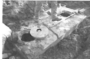
Repair Tank 4-16-19 140 Poi
