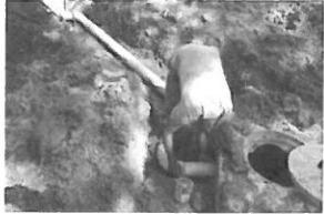
Repair Tank 4-16-19 140 Poi
