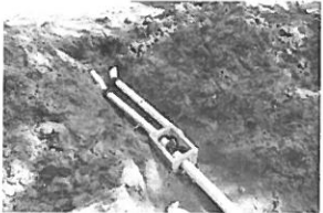
Repair Tank 4-16-19 140 Poi
