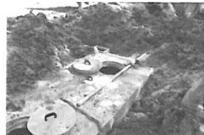
Repair Tank 4-16-19 140 Poi
