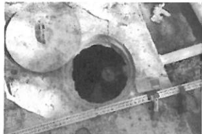
Repair Tank 4-16-19 140 Poi
