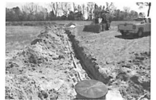
Hwy 27 & SR1409 Hodges Ch.
