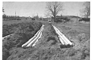
Hwy 27 & SR1409 Hodges Ch.
