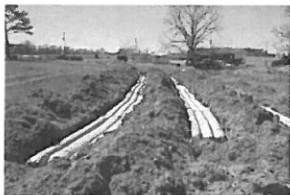
Hwy 27 & SR1409 Hodges Ch.
