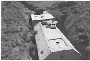
Hwy 27 & SR1409 Hodges Ch.
