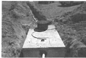
Hwy 27 & SR1409 Hodges Ch.
