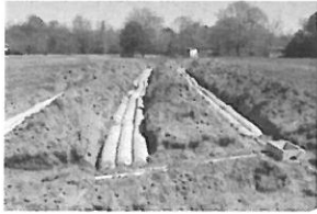
Hwy 27 & SR1409 Hodges Ch.
