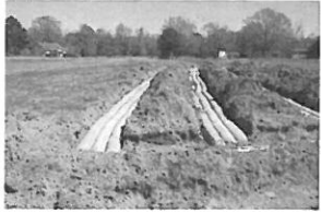
Hwy 27 & SR1409 Hodges Ch.
