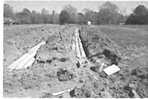
Hwy 27 & SR1409 Hodges Ch.
