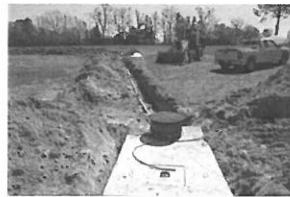
Hwy 27 & SR1409 Hodges Ch.
