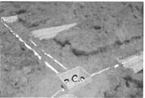
Hwy 27 & SR1409 Hodges Ch.
