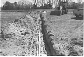
Hwy 27 & SR1409 Hodges Ch.
