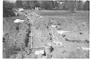
Hwy 27 & SR1409 Hodges Ch.
