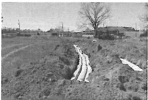
Hwy 27 & SR1409 Hodges Ch.
