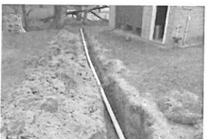
lozynski Repair 10-25-18 Gar
