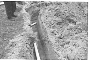
lozynski Repair 10-25-18 Gar
