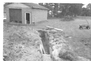
lozynski Repair 10-25-18 Gar
