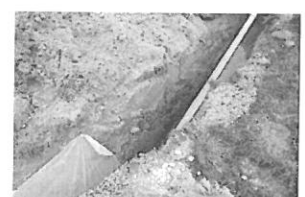
lozynski Repair 10-25-18 Gar
