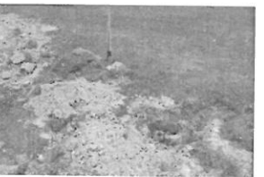
lozynski Repair 10-25-18 Gar
