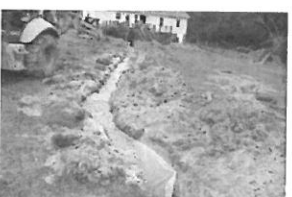
lozynski Repair 10-25-18 Gar
