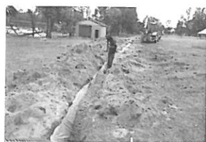
lozynski Repair 10-25-18 Gar
