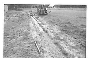
lozynski Repair 10-25-18 Gar
