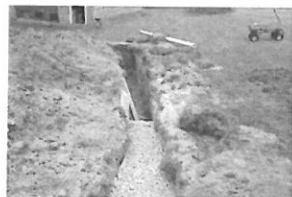
lozynski Repair 10-25-18 Gar
