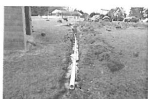
lozynski Repair 10-25-18 Gar
