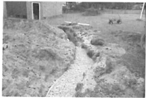
lozynski Repair 10-25-18 Gar
