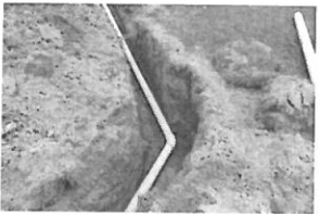
lozynski Repair 10-25-18 Gar
