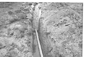
lozynski Repair 10-25-18 Gar
