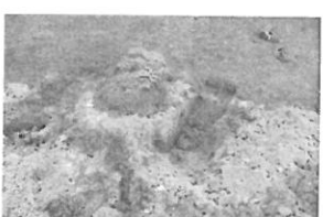
lozynski Repair 10-25-18 Gar
