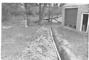
lozynski Repair 10-25-18 Gar
