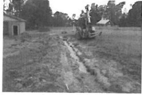
lozynski Repair 10-25-18 Gar
