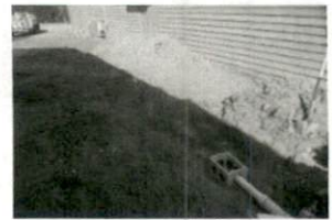
man Repair SR1538 Mabry RI
