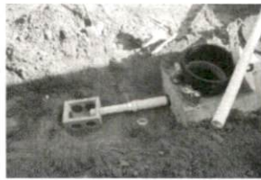
man Repair SR1538 Mabry RI
