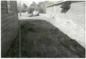
man Repair SR1538 Mabry RI
