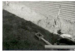
man Repair SR1538 Mabry RI
