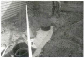
man Repair SR1538 Mabry RI
