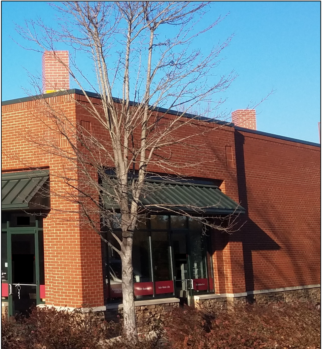
Exhibit D – Faux Chimney Example
