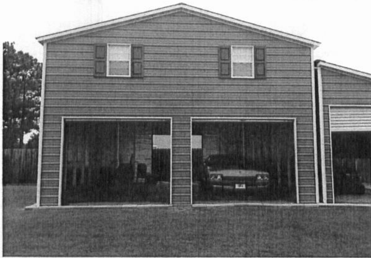
Exhibit A: The exterior of the building was constructed in accordance with plans provided by carport installer.
