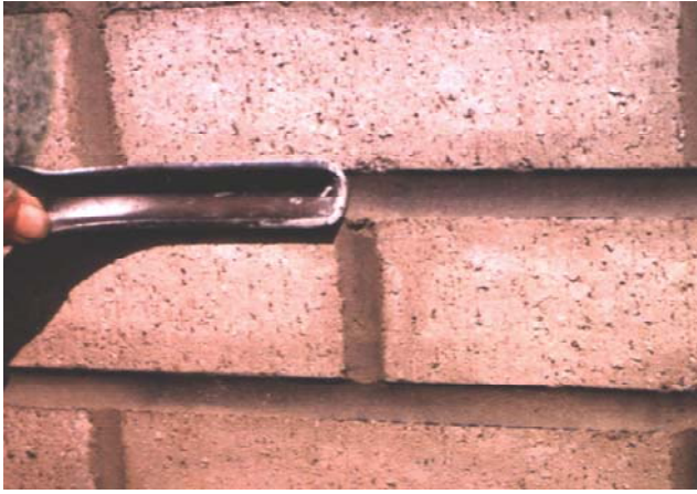
Photo 4 Concave Mortar Joints
