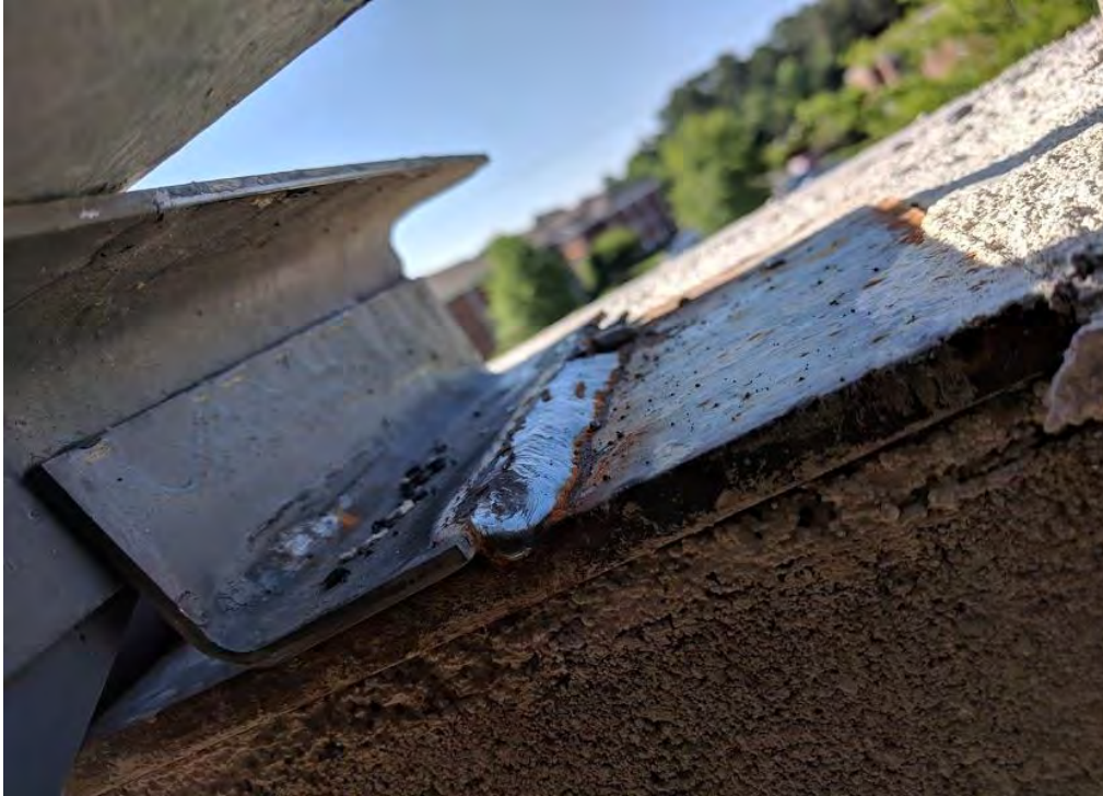
Joist End Weld
