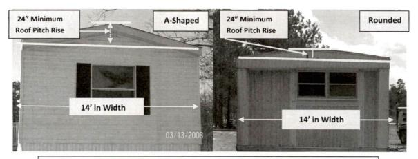
Note: Most rounded roofs will not meet the roof pitch requirement as illustrated.
