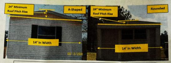
Note: Most rounded roofs will not meet the roof pitch requirement as illustrated.
