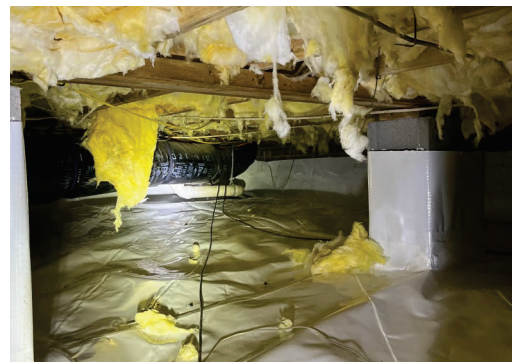
Picture 2 – Typical crawlspace conditions and first-floor framing
