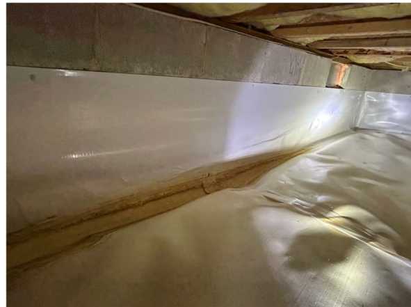
Picture 2 – Typical crawlspace conditions and first-floor framing
