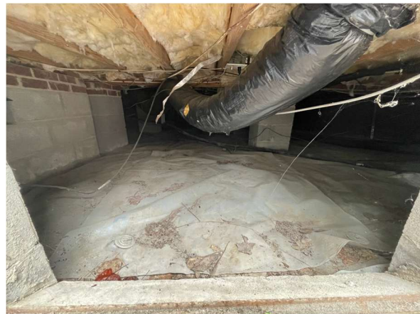
Picture 2 – Typical crawlspace conditions and first-floor framing
