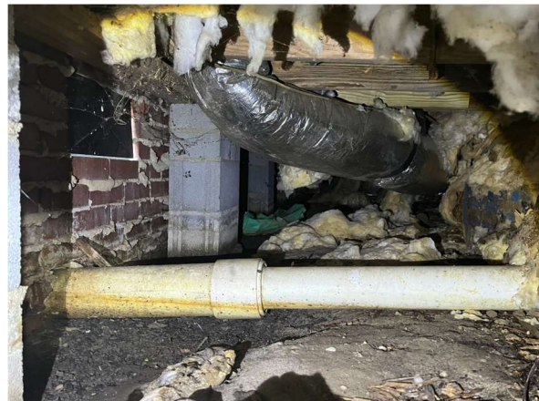
Picture 2 – Typical crawlspace conditions and first-floor framing
