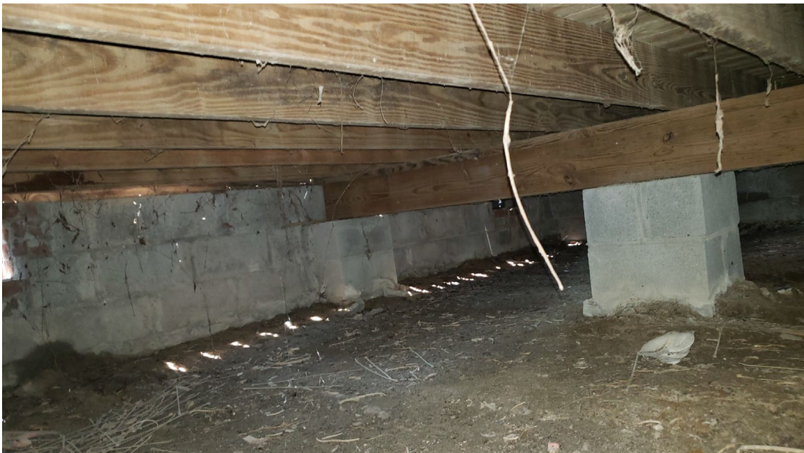
Item 1) Examples of existing porch foundation (floor framing to be removed per conversation with homeowner)
