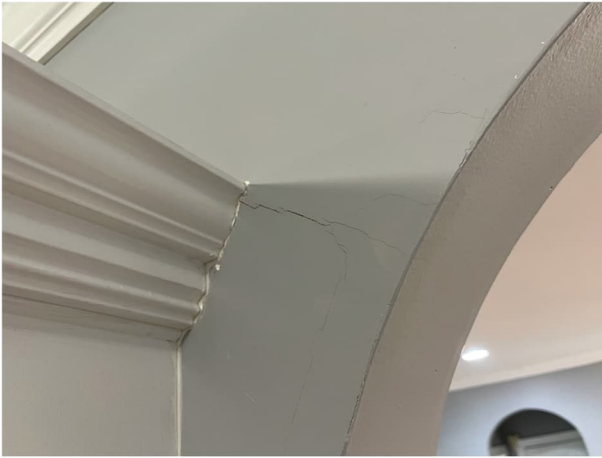
Picture 5 – Drywall cracks
