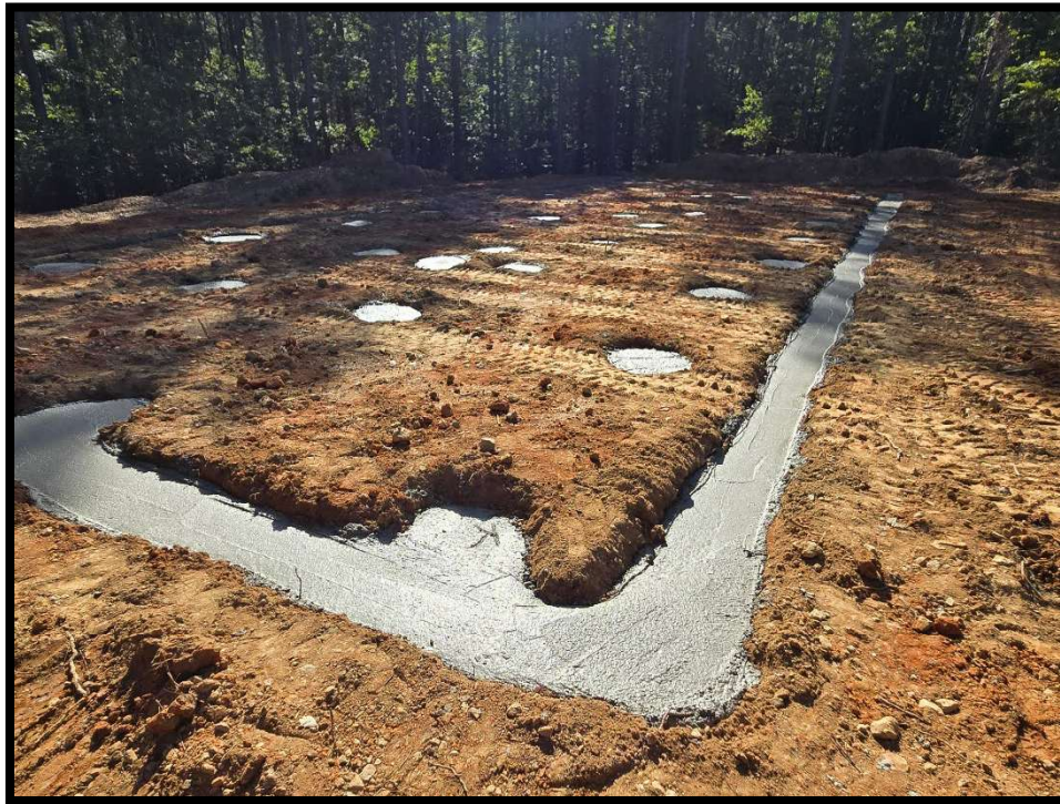
(Pier Foundation with Concrete)
