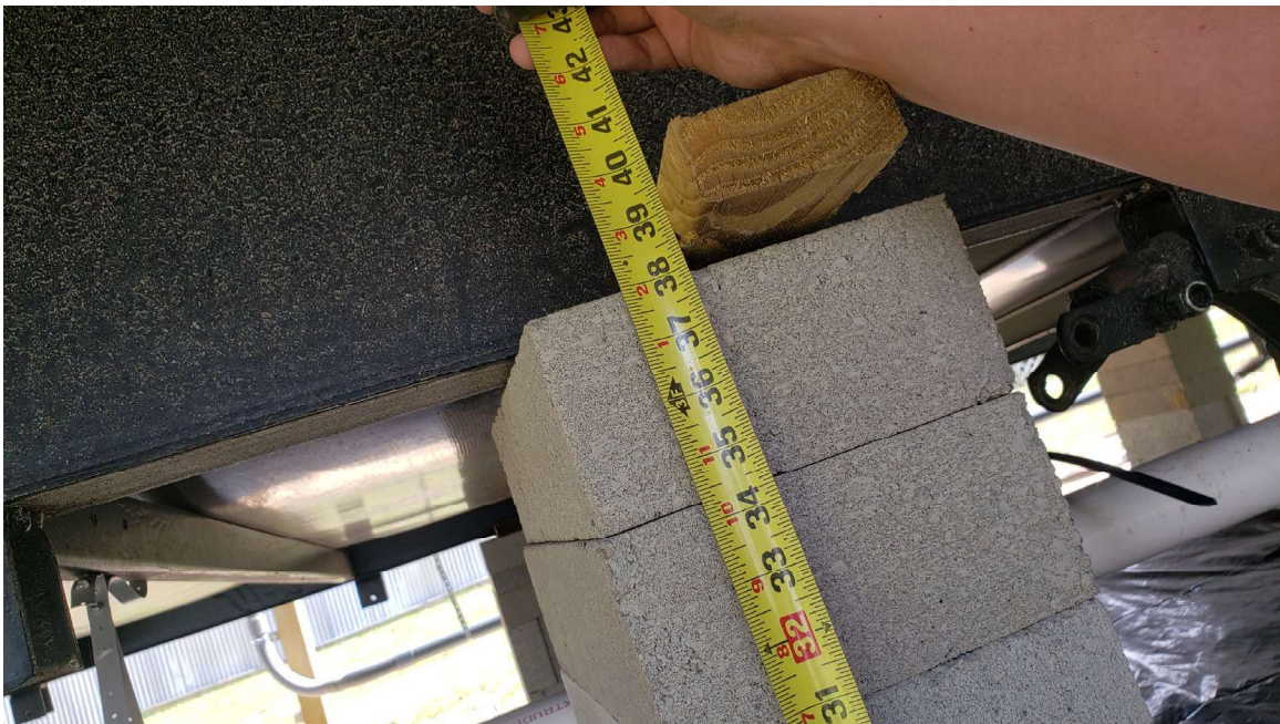
Example of 8" x 16" CMU pier over 36" in height above grade
