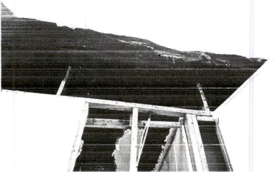
Picture 4 - Example of fire damaged roof truss
