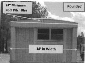
Note: Most Rounded Roofs Will Not Meet The Roof Pitch Requirement As Illustrated. The Measurement From The Peak Of The Roof To The Base Line Of The Roof Must Be 12" For Every 7' Of Total Width Of The Home. (Ex: 14' Wide Home = 24" Roof Rise)
