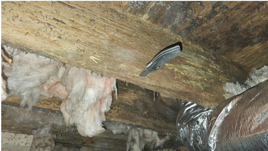
Picture 6 – An example of a deteriorated joist
