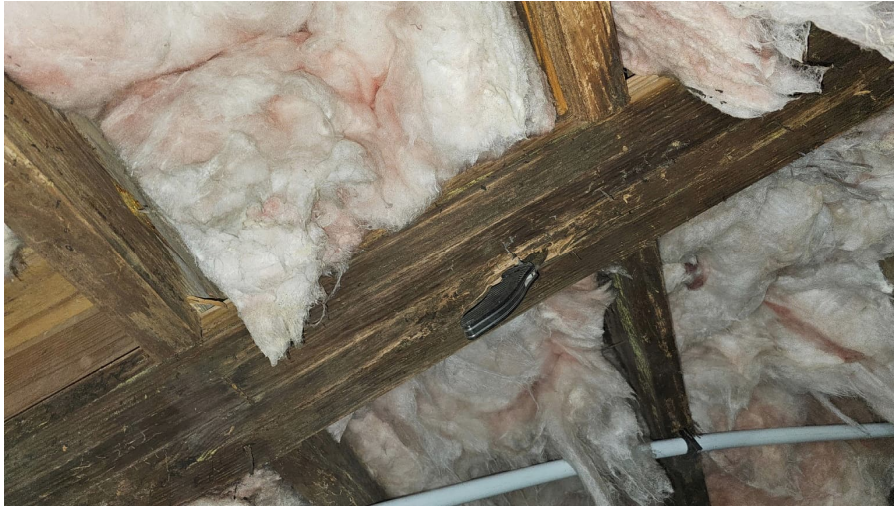
Picture 3 – Example of a deteriorated girder
