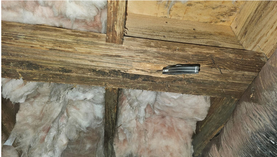
Picture 5 – An example of a deteriorated girder.
