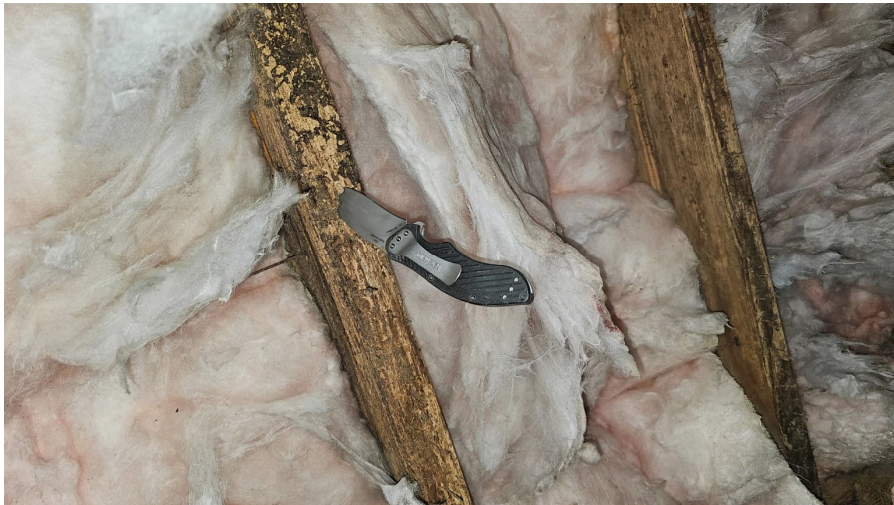
Picture 4 – An example of a deteriorated joist
