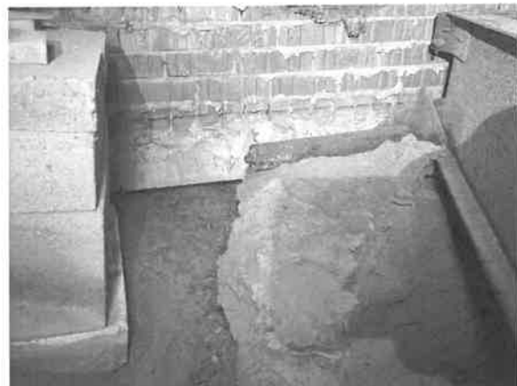
Picture 6 – Evidence of Water Intrusion
