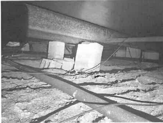
Picture 3 – Leaning and Failed Foundation Elements
