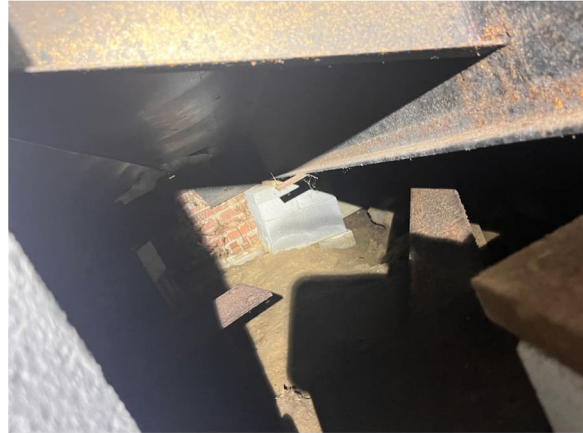
Picture 4 – Leaning Foundation Elements
