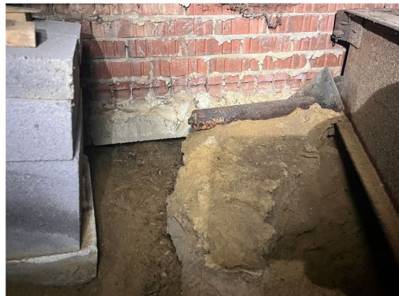
Picture 6 – Evidence of Water Intrusion
