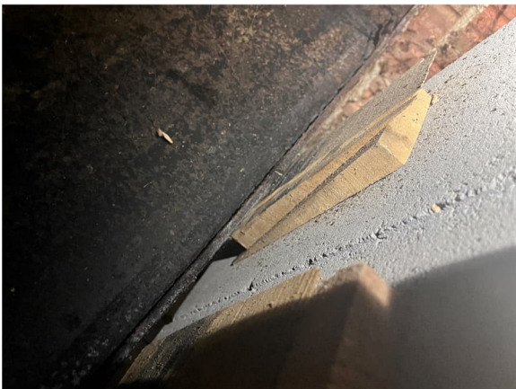
Picture 5 – Pier out of Contact with Chassis Beam
