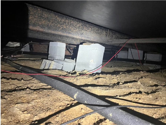
Picture 3 – Leaning and Failed Foundation Elements
