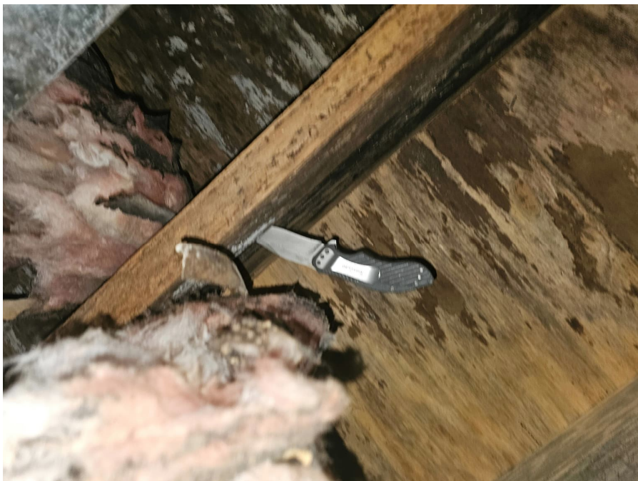
Picture 4 – Example of deteriorated joist
