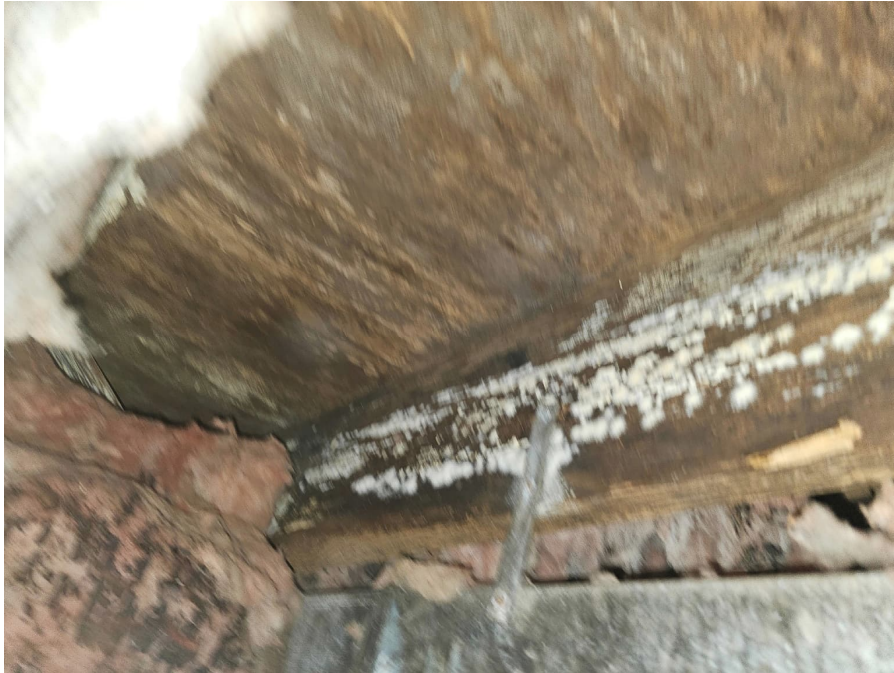
Picture 3 – Example of deteriorated joist
