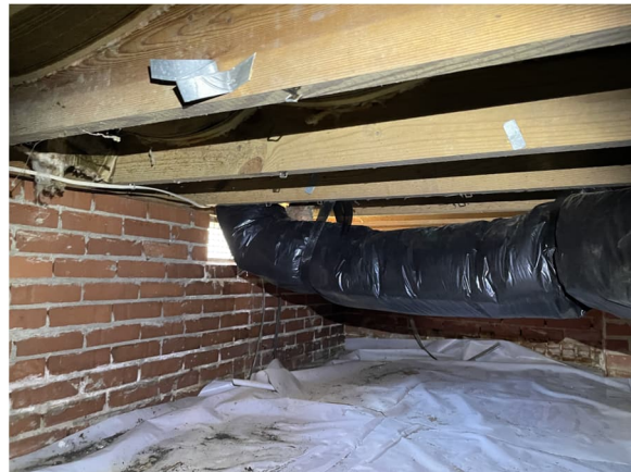
Picture 2 – Example of 1 st floor framing
