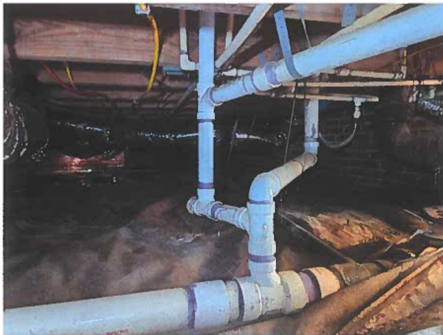
Picture 2 – Left rear area of crawlspace to be stabilized
