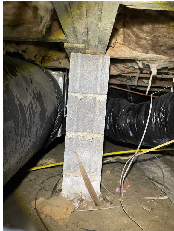
Picture 4 – Typical Interior Foundation Element
