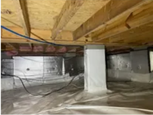
Picture 3 – Existing Foundation System and Typical First Floor Framing
