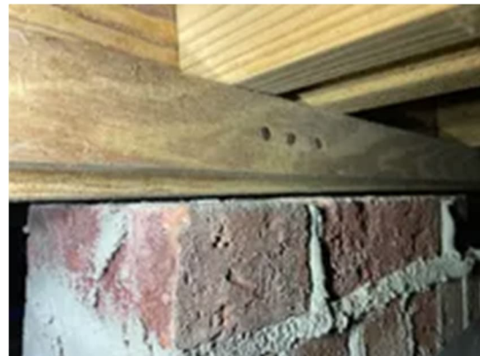
Picture 6 – Out-of-Contact Pier
