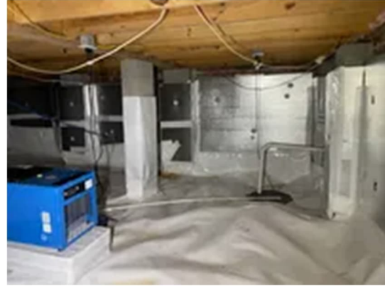
Picture 4 – Existing Crawlspace (Closed Crawlspace System)
