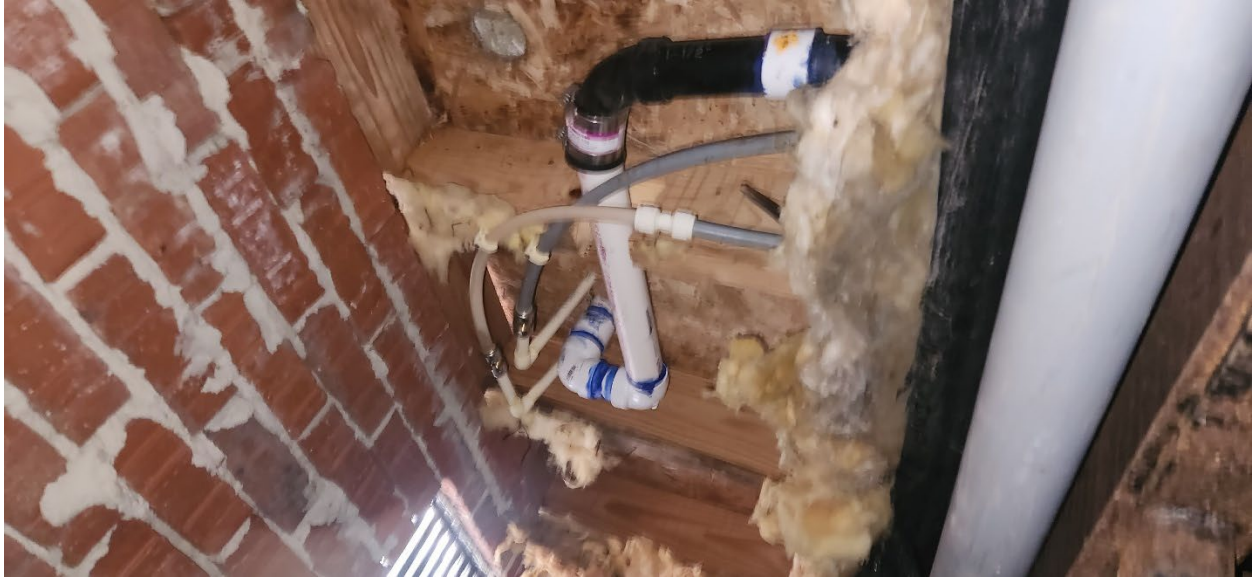
Notched Floor Joist
