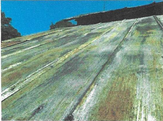
(19A) – Roof Coating Chrysotile 3%
