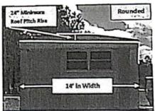
Note: Most Rounded Roofs Will Not Meet The Roof Pitch
