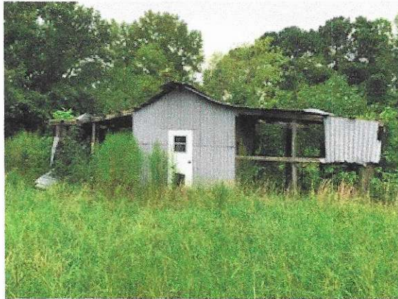
Shop W/ Attached Lean-Too's
