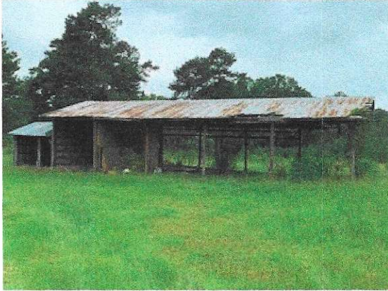
5 Bay Equipment Shelter
