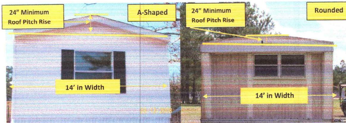
Note: Most rounded roofs will not meet the roof pitch requirement as illustrated.
