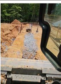
Repair for soft soils in drain line repaired with washed stone
