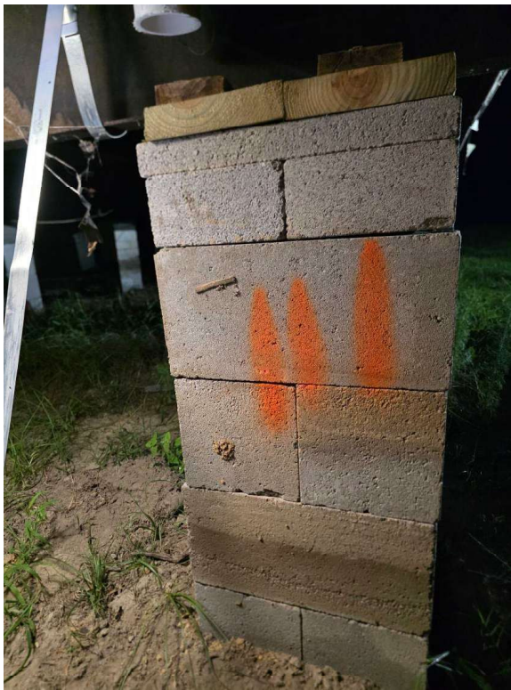
Examples of piers in correct orientation per previous report
