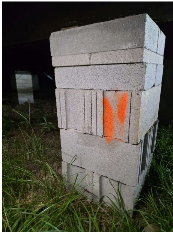
Examples of piers in correct orientation per previous report
