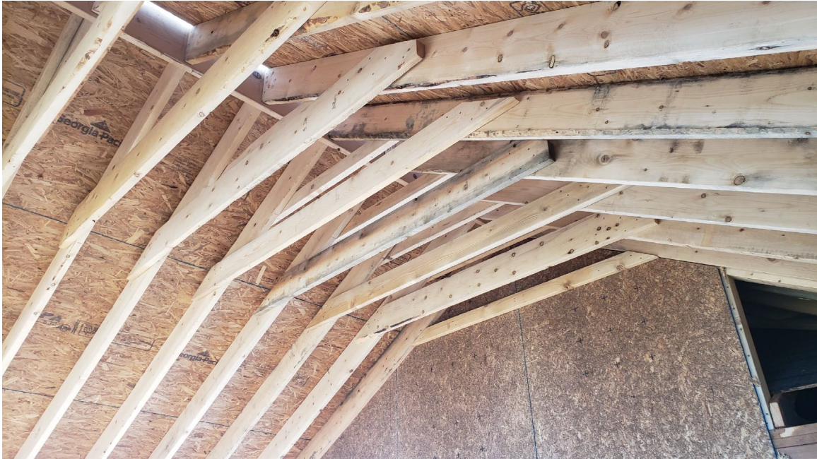
Example of existing collar ties
