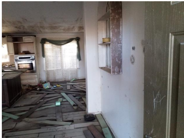
002A, 002 - Gypsum Wallboard Joint Compound, Living Room, Main Floor
