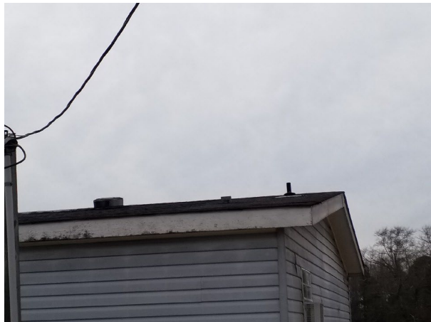
001B, 001 - Roofing, Composite Shingle, Exterior, Main Floor
