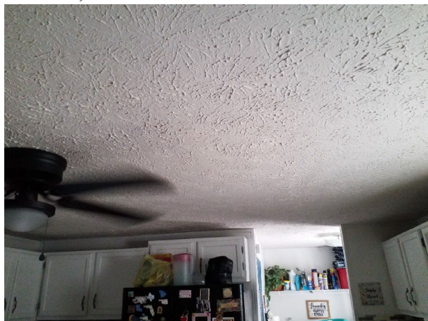
002B, 002 - Textured Ceiling, Kitchen, Main Floor
