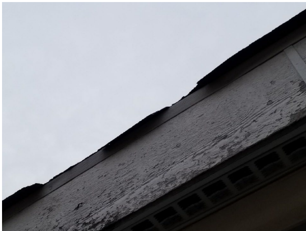
001A, 001 - Roofing, Composite Shingle, Exterior, Main Floor
