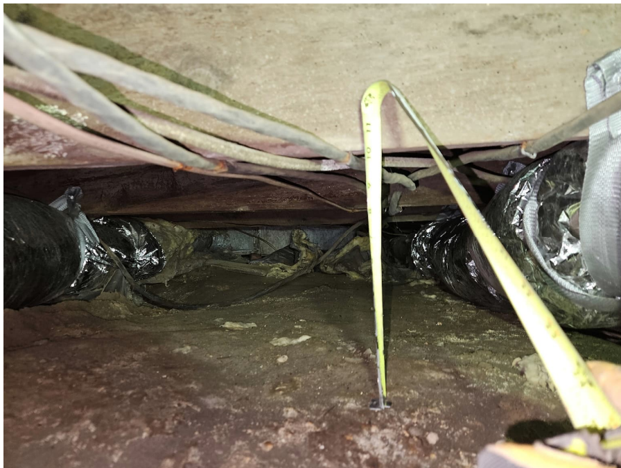
Picture 4 – Inadequate clearance
