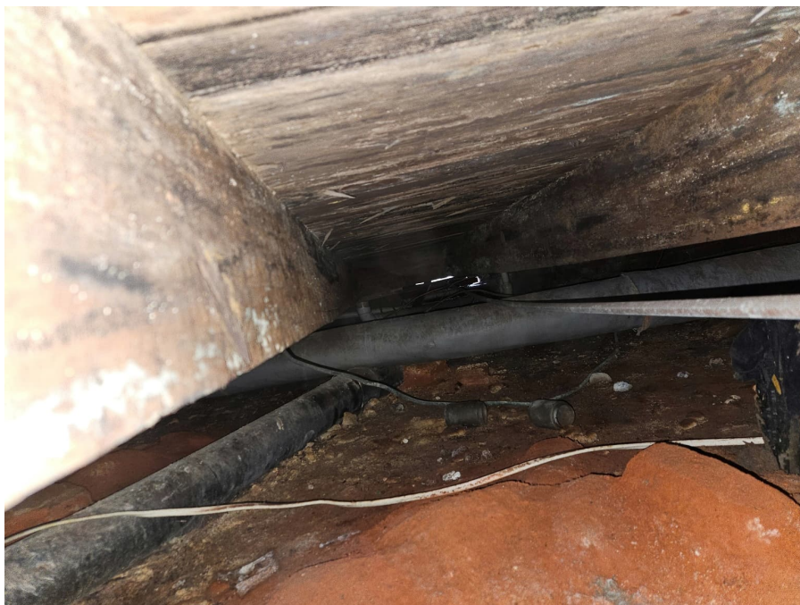
Picture 6 – Deteriorated joist
