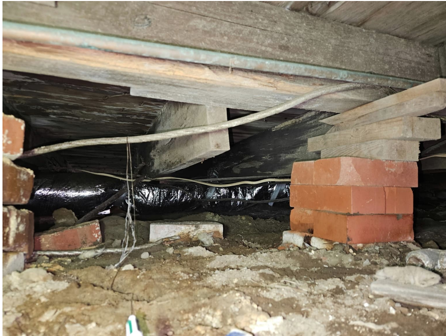
Picture 3 – Inadequate brick pier
