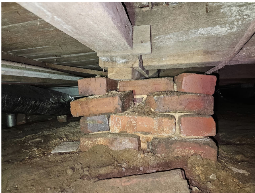
Picture 2 – Inadequate brick pier
