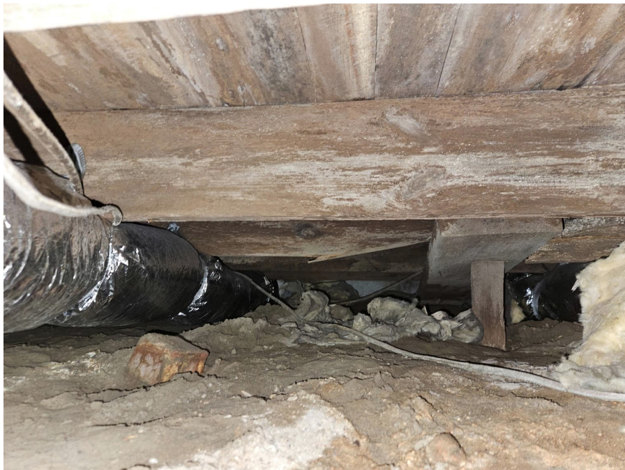
Picture 8 – Deteriorated joists past inadequate clearance
