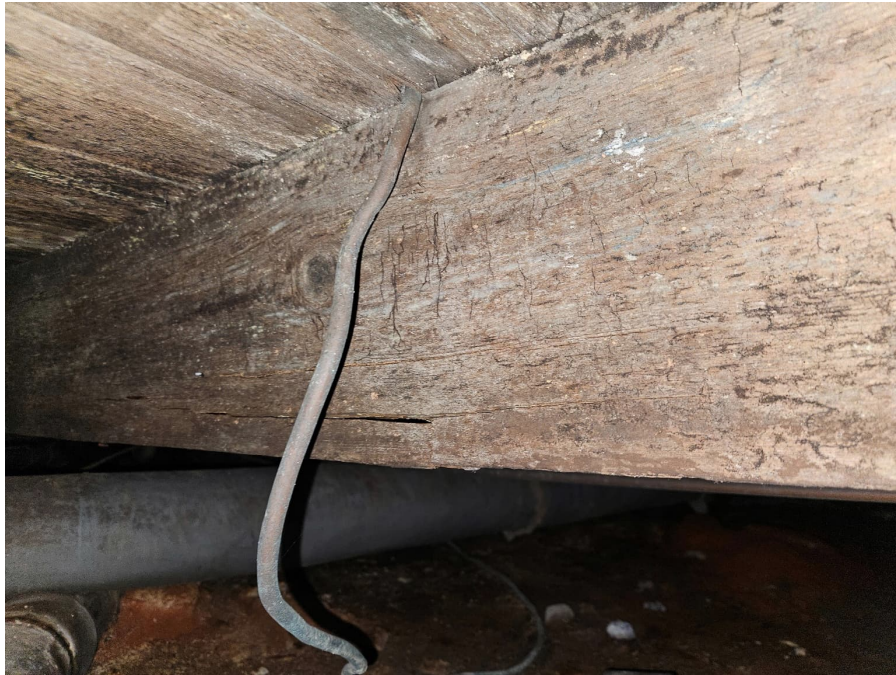
Picture 5 – Deteriorated joist
