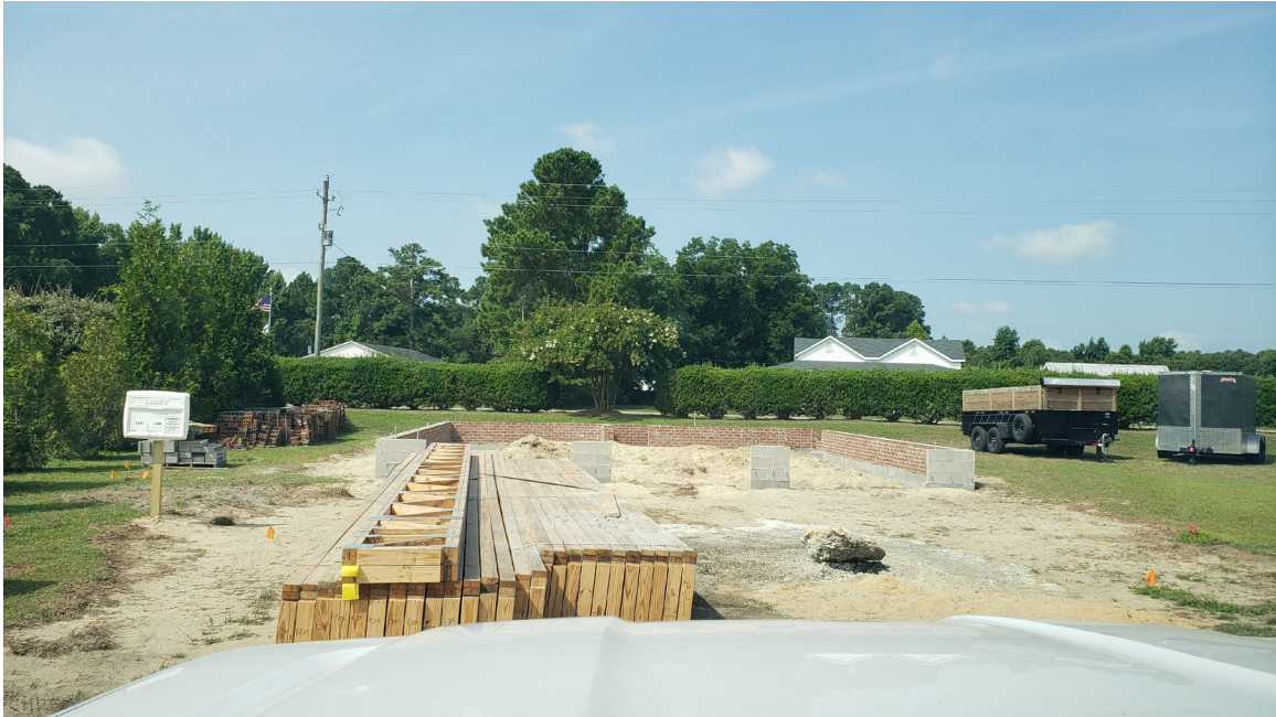
Existing site conditions
