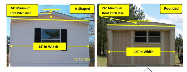
Note: Most Rounded Roofs **Will Not** Meet The Roof Pitch Requirement As Illustrated. The Measurement From The Peak Of The Roof To The Base Line Of The Roof Must Be 12" For Every 7' Of Total Width Of The Home. (Ex: 14' Wide Home = 24" Roof Rise)
