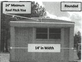
Note: Most Rounded Roofs Will Not Meet The Roof Pitch
