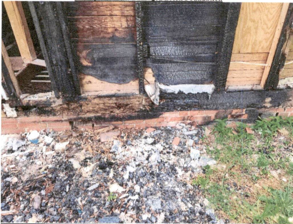
Example of Heat Damaged Brick Foundation
