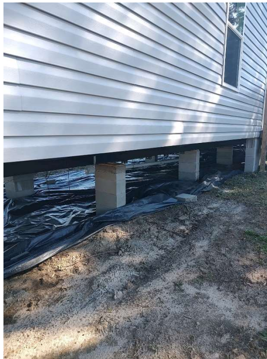
Site Photo 1: Tallest pier above grade, (double-stacked CMU w/ lateral bracing)
