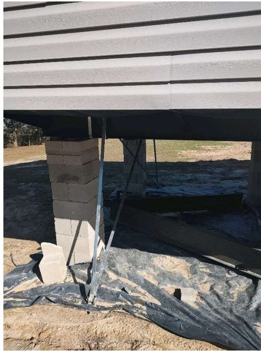
Site Photo 1: Tallest pier above grade, (double-stacked CMU w/ lateral bracing)
