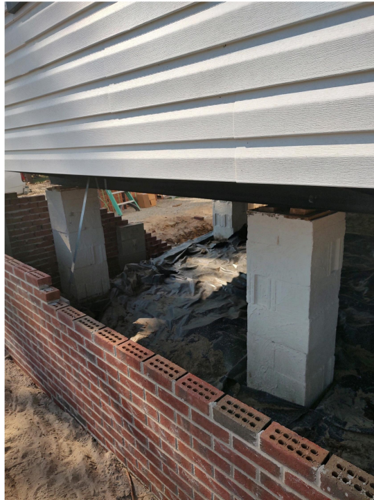
Photo 1: Typical pier placement/ orientation at high side
