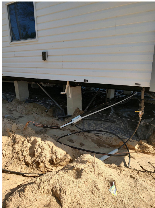
Photo 2: Typical pier placement/ orientation at low side
